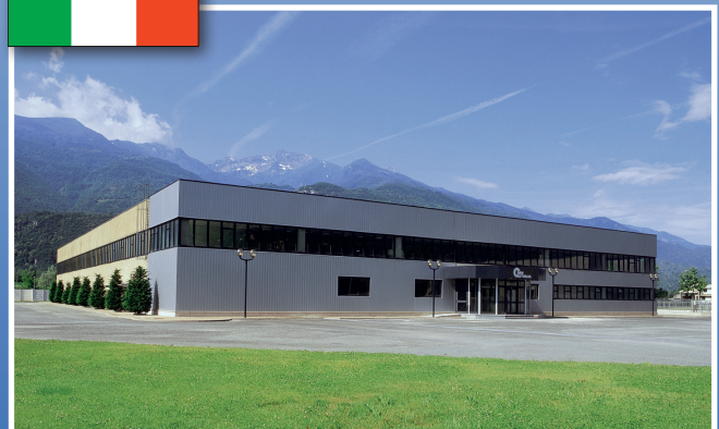
AUTOBLOK manufacturing plant Caprie-Torino
