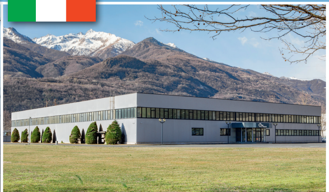
AUTOBLOK manufacturing plant Caprie-Torino
