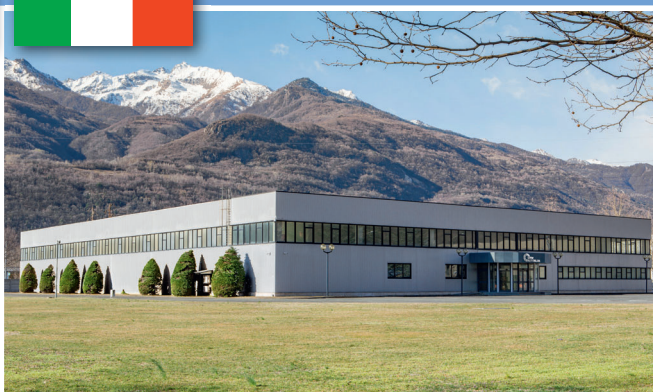
AUTOBLOK manufacturing plant Caprie-Torino
